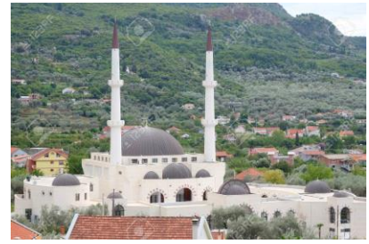
Mosque in Bar, Montenegro
